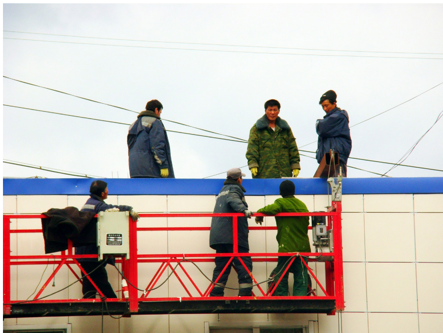
North Koreans working on a construction site in Vladivostok.
