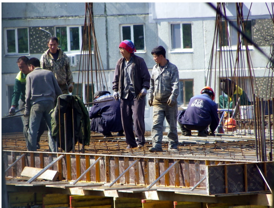
North Koreans working on a construction site in Vladivostok.
